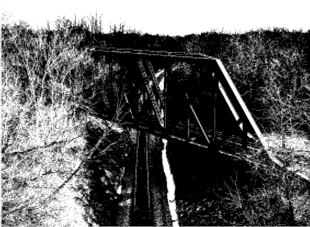
Plate 7. View of the Southern Railroad Skew Bridge, BE 653, from Walton Nicholson Road facing north
