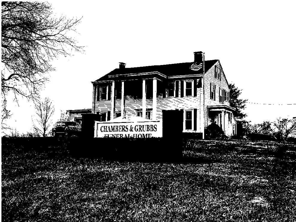
Plate 1. View of the Chambers and Grubb Funeral Home at 118 Chambers Road, BE 536, from Chambers Road facing north
